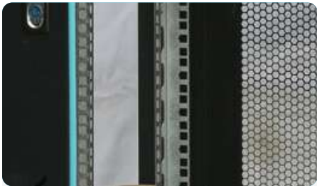
加厚立梁 The vertical beam was thickened
